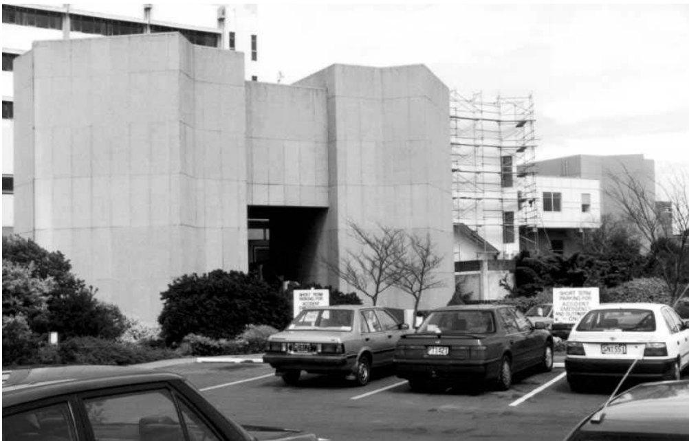
'Twin tower' entrance to Palmerston North Hospital. The two 'towers' were for supervoltage therapy units, a Theratron-80 Co-60 unit, and the Siemens betatron (in use 1974). These are at first-floor level; also, a corridor can be seen off to the right, leading to the later addition of a Varian 21C linac in a matching 'tower' building
